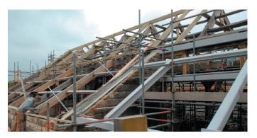
But the barn was in distress; a few of the oak beams were dangerously rotten due to exposure to the elements at times, one side wall was leaning out. Despite many attempts to buttress up the walls and to keep the metal sheeting roof in place, its days were limited. The barn was now a Grade Two listed building, but the funds were not there to save it from disrepair and ultimate collapse.
